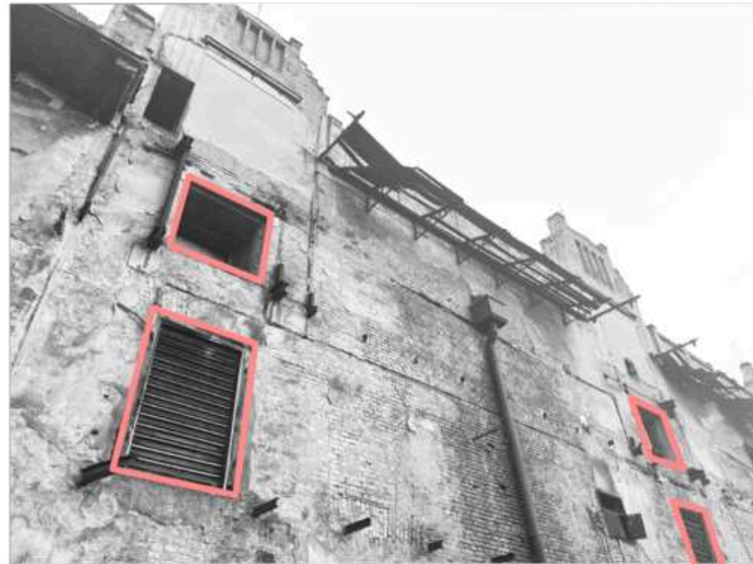
14 Ledárny - elevator shafts for ice transportation
